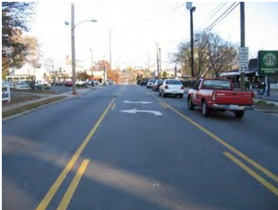
Figure 6. Example of two-way center turn lane. Photo credit FHWA.
